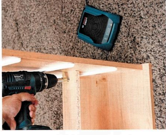
▲ ...and easily in reach for driving in the fixings as needed
